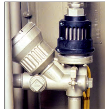
The Millennium pneumatic remote control valve combines inlet and outlet functions.
