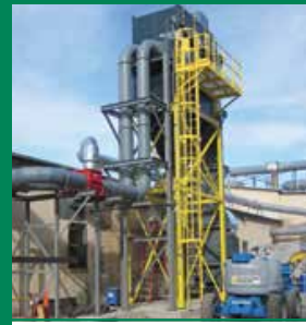
Heat Exchanger for Exhaust Gas that Cannot be Recirculated
