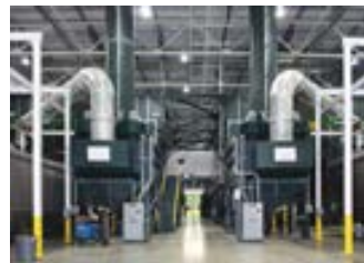
GS60 on blasting at National AL Railcar
